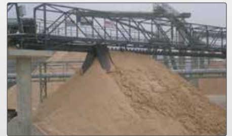
fines conveyor with spreading auger
