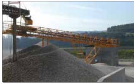
lattice bridge with belt conveyor
